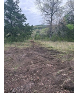
Back fill of the overflow pipe
